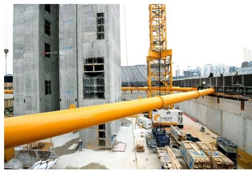
McGee were able to provide significant value to the Client through the use of Slipform for the core, this shortened the programme, and we completed the exercise ahead of schedule.
